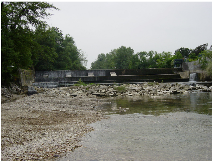
Fig. 3: River dam at low river discharge ( 9 \text{ m}^3/\text{s} ; 16.06.2006). Note, as evidence for the subsidence of the dam structure, that the crest is only overflowed on its left side (a perspective is given in Fig. 1)
