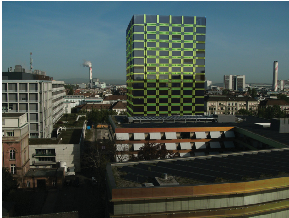
Figure 83: Hybrid image showing the new building in its environment, using an omnidirectional panorama as the light source for the scene (Image: F. Müller)
