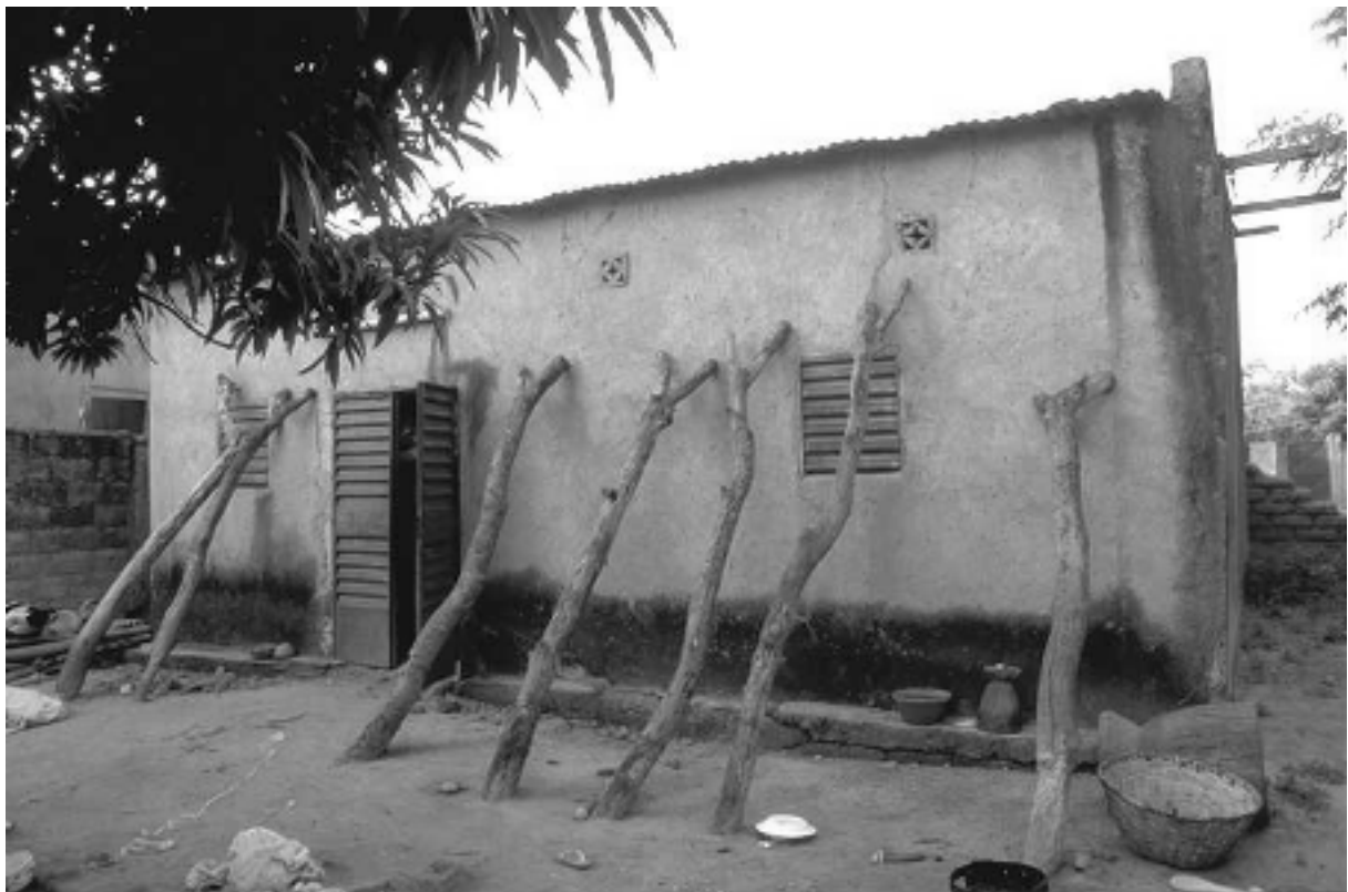
Photo 15: House constructed with adobes and stabilized with trunks after the rainy season
