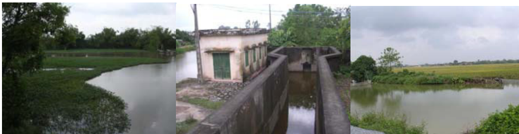
Photo 3.1 Nhue River and water pumping station for irrigation to the fields in Nhat Tan and Hoang Tay communes, Northern Vietnam
