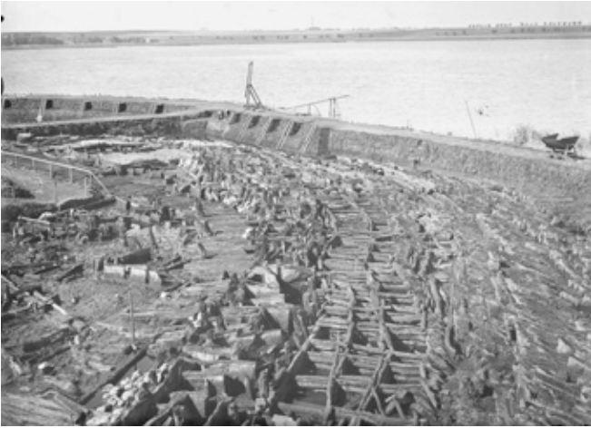
Figure 21: Breakwater palisade and encircling rampart of the Biskupin fortified settlement. The breakwater is visible on the right of the image, consisting of angled piles driven into the ground angled towards the settlement (image: the Poznan Archaeological Museum http://www.muzarp.poznan.pl/muzeum/muz_pol/Arena/Biskupin/gal_eng.html ).
