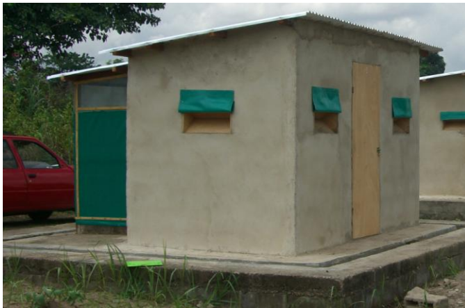
Figure 5.1: Experimental huts used in the study located in the M'Bé site, near Bouaké in central Côte d'Ivoire. The experimental huts comprised a sleeping room and a veranda. The walls of the room were either made of concrete bricks coated with cement (A) or wood structures coated in dry mud – locally called “banco” (B).
