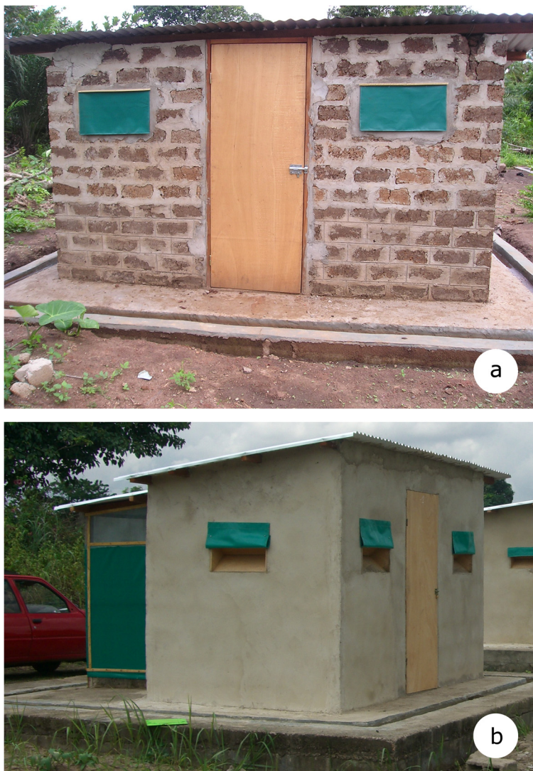
Figure 1 Experimental huts used in the study located in the M'Bé site, near Bouaké in central Côte d'Ivoire. The experimental huts comprised a sleeping room and a veranda. The walls of the room were either made of concrete bricks coated with cement (a) or wood structures coated in dry mud – locally called banco (b).
