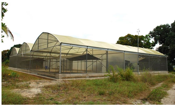
Figure 2 Semi-field system. The walls and the roof of the semi-field system (SFS) are made of metal frames and fiberglass netting material. The SFS has two sections separated by heavy-duty polyurethane. Each of these sections contains one experimental unit.
