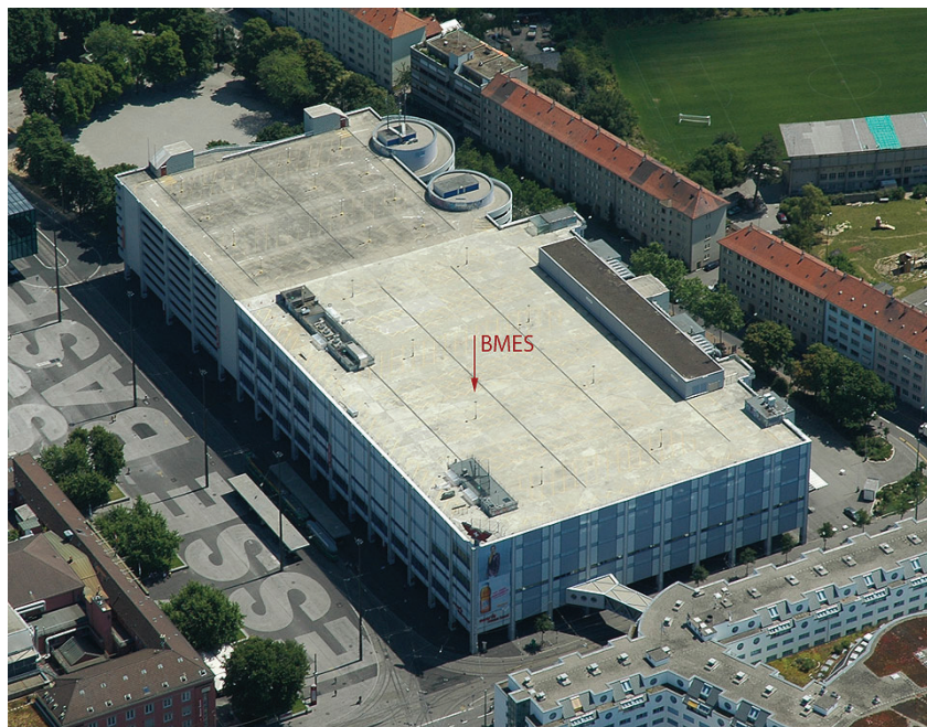
Fig. A.4: Aerial view of the concrete roof from West at the Messe site (U3) (Photo by Roland Vogt, 16.7.2004)
