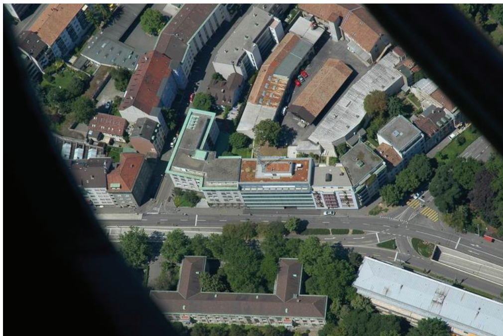
Fig. A.3: The Klingelbergstrasse site with the measurement tower located on the roof of the new institute. July 16, 2004 (Photo by R. Vogt).
