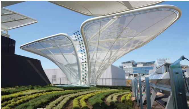
Figure 1.3: Examples for integrated OPV application. The picture shows the german pavillon at the EXPO world exhibition 2015 in Milan, equipped by Belectric OPV (Ref. [54]).
