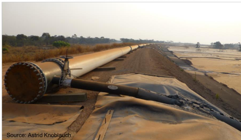
Tailings dam, Trident project, Kalumbila Copper Mine, Zambia
