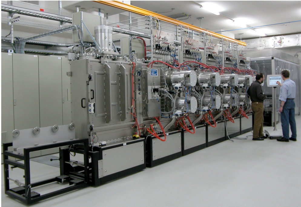
Figure 4.3: Laboratory in-line plant of the Glas Trösch AG. The glass panes enter the in-line plant on the right side and are moved vertically past the different cathodes for the deposition of the different layers. Each cathode contains a different material. The whole in-line plant has five cathodes.
