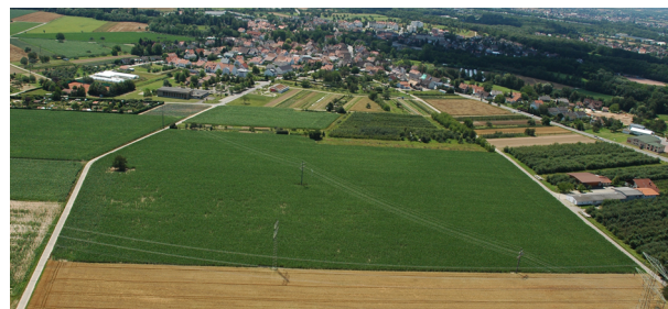
Figure 3.2: Aerial view of the site southbound (photograph by R. Vogt).
